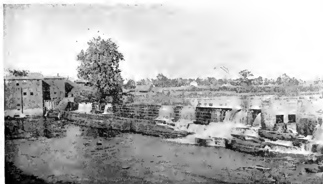
A View of the Dam—Chicopee Falls
